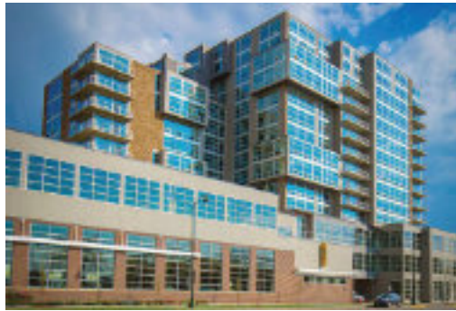
The new office is in the Galaxie High Rise Development on East Washington Avenue in Madison, WI.
